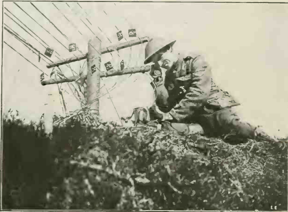
A British "Tommy" Repairing Telephone Lines Near the Battle-Front. Note the Short Poles in Use.
